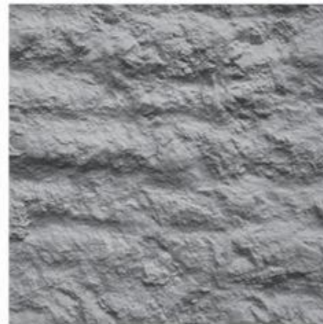
CSP 9 HEAVY SCARIFICATION
