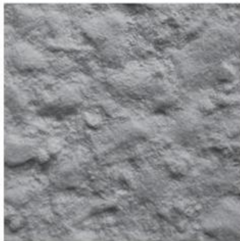
CSP 7 HEAVY ABRASIVE BLAST
