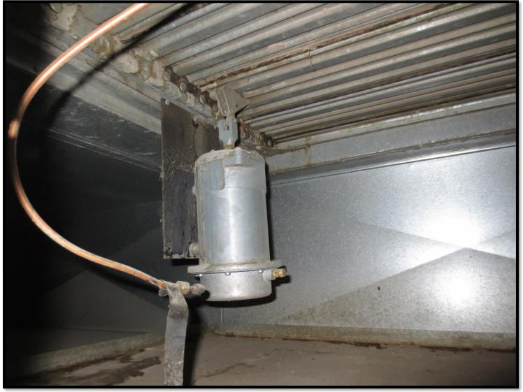
Elbow insulation not installed
