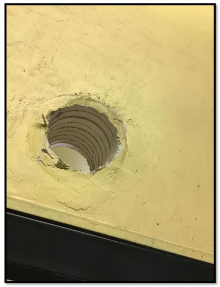
Wall was not cleaned after core drilling
