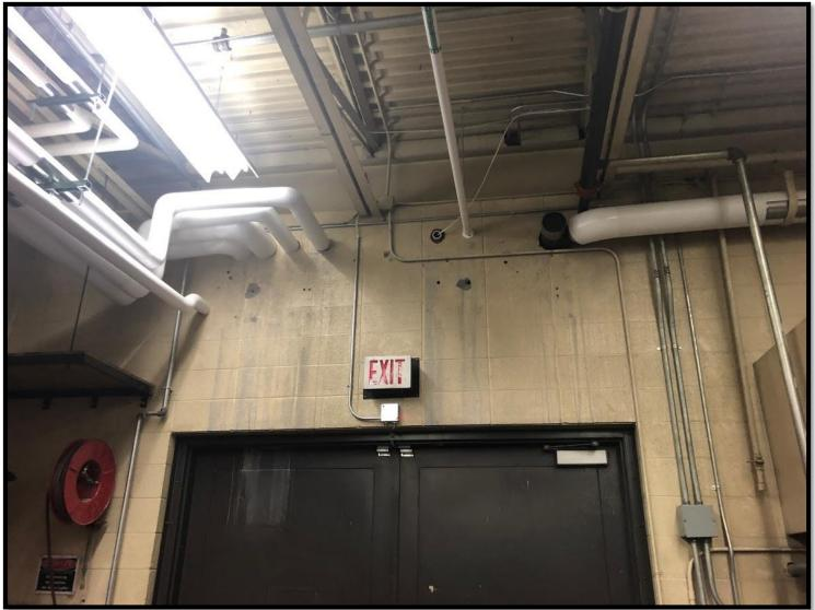
Failed to remove dust cover from ductwork
