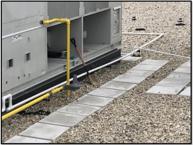
Disconnect switch not installed
